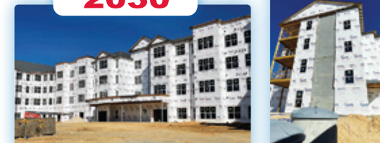
New Construction at Haven at Palmer Pointe
