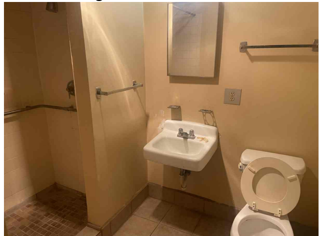
Bathroom – 1 Bedroom Unit
