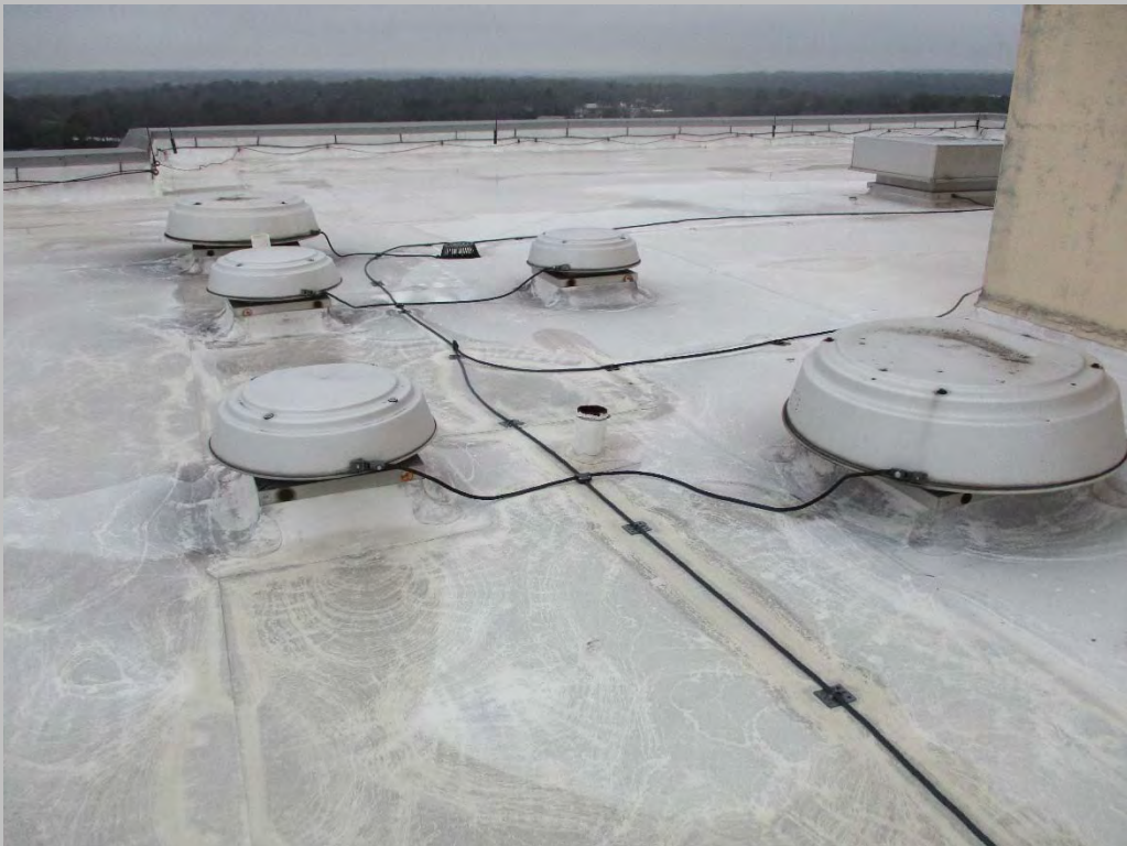
Building membrane roof
