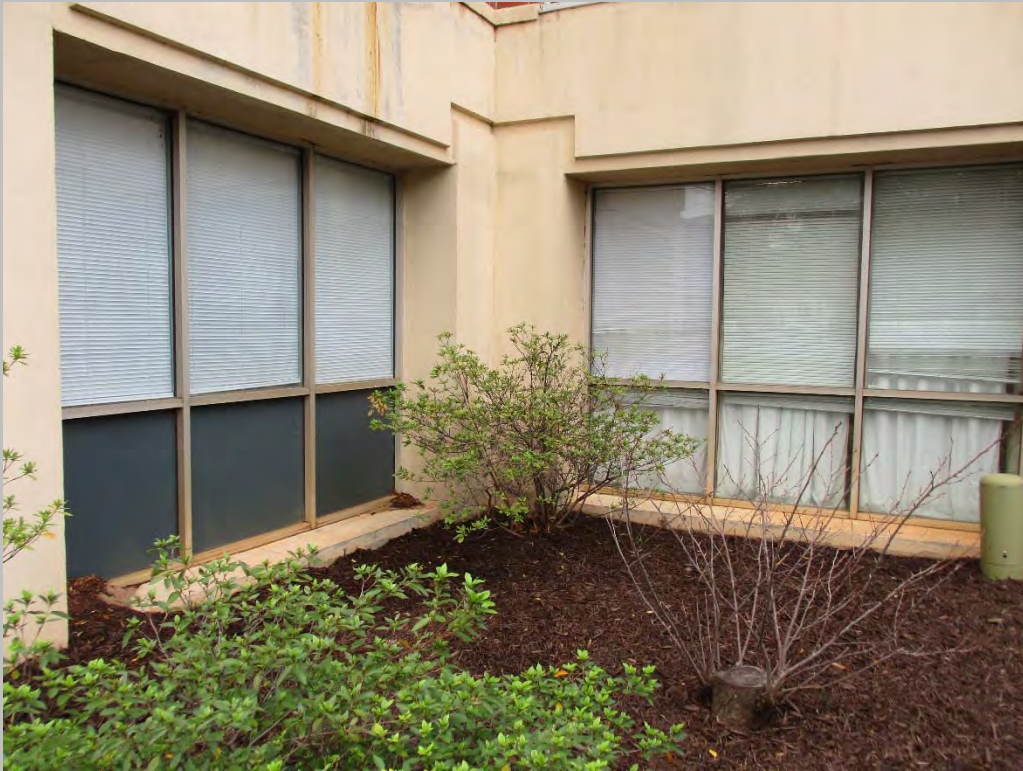
Typical ground-level glass storefront window assemblies
