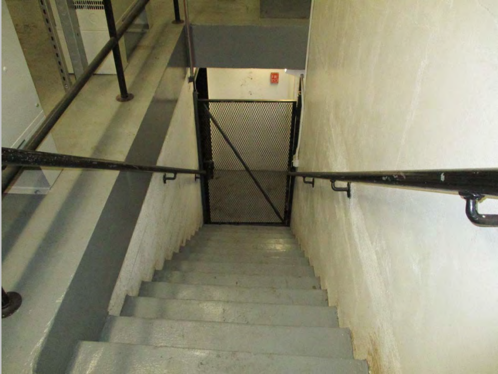
Typical building stairwell
