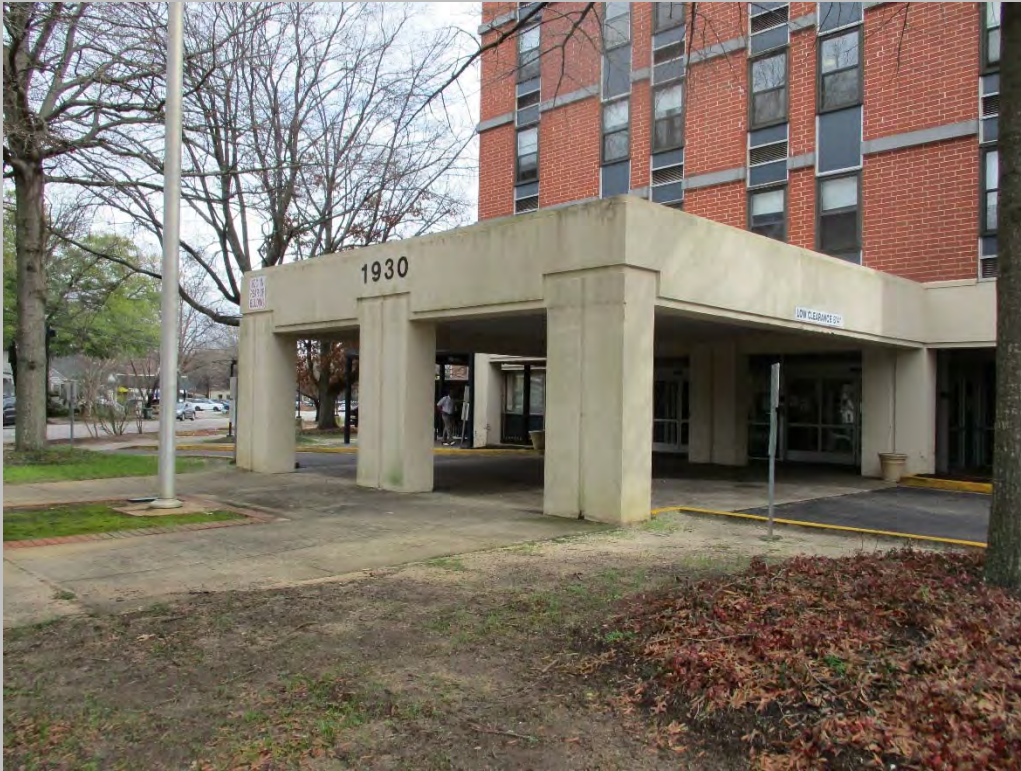
Porte cochere at the main entrance
