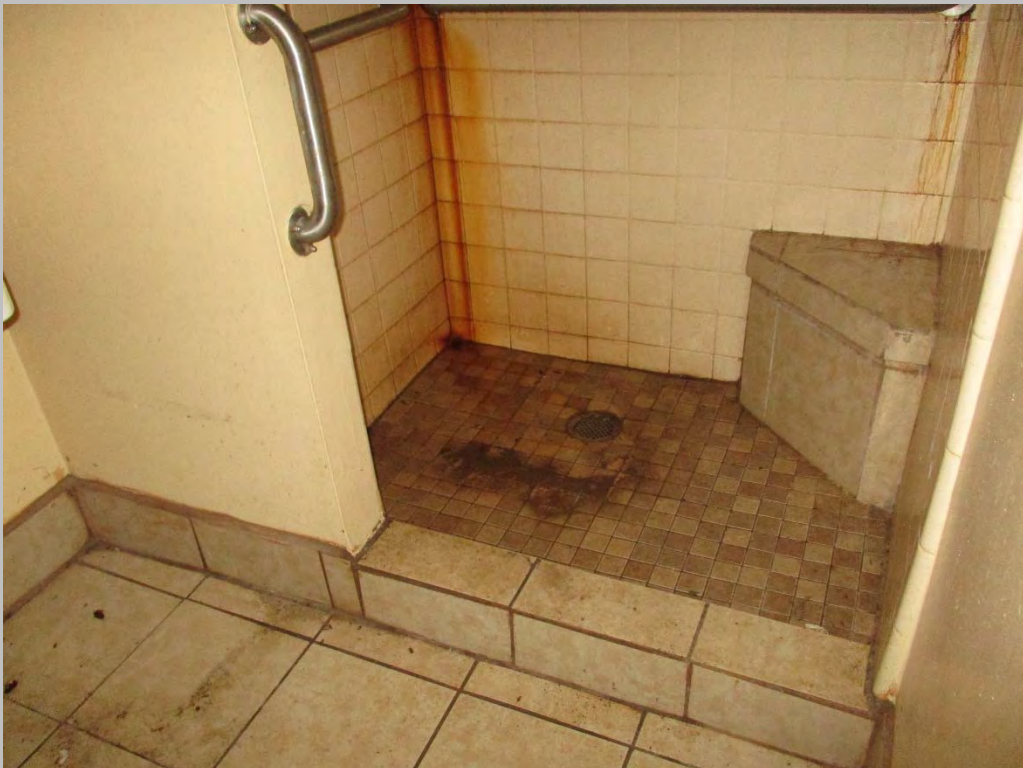
Typical dwelling unit bathroom
