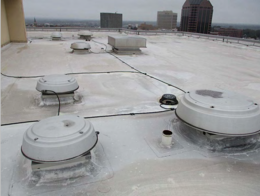
Building membrane roof
