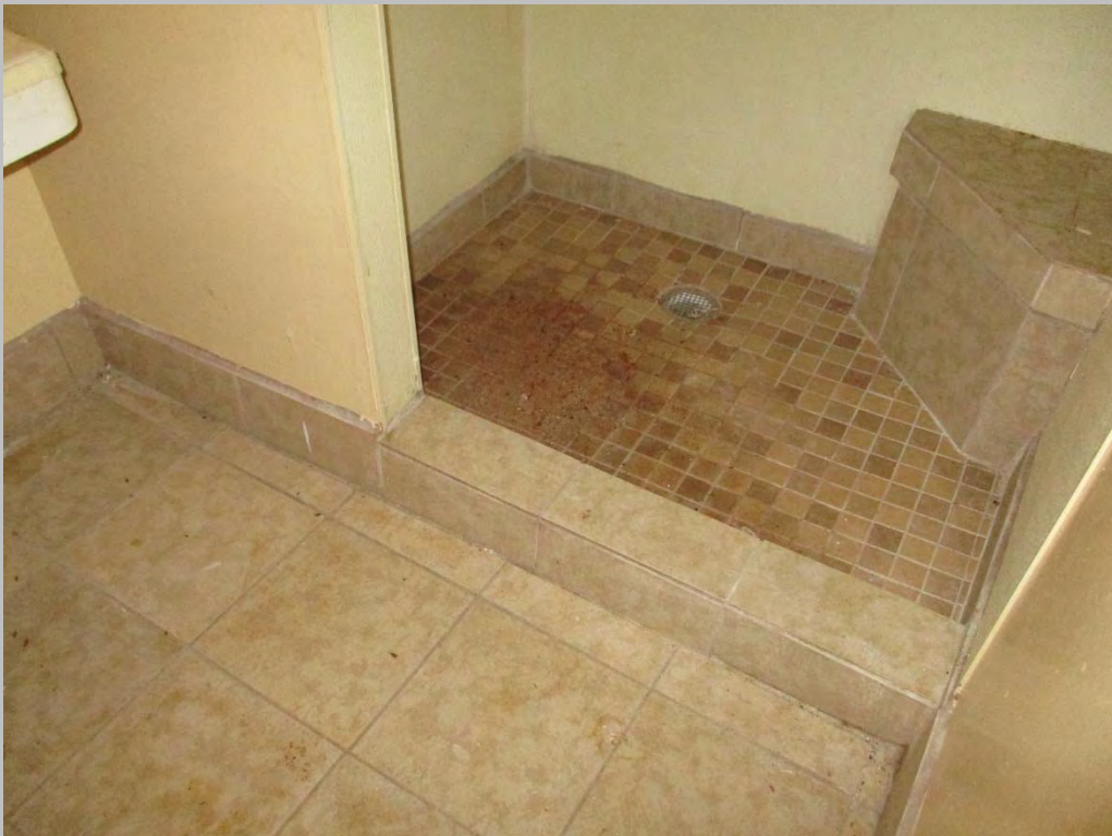
Typical dwelling unit bathroom
