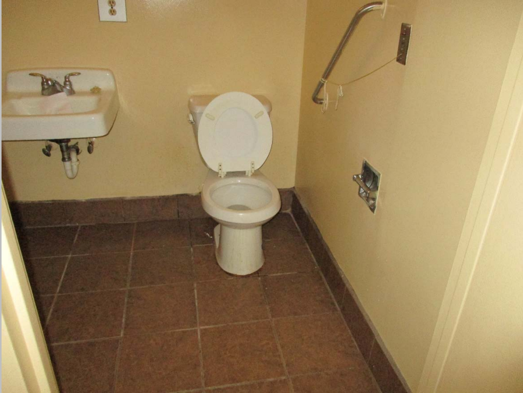
Typical dwelling unit bathroom
