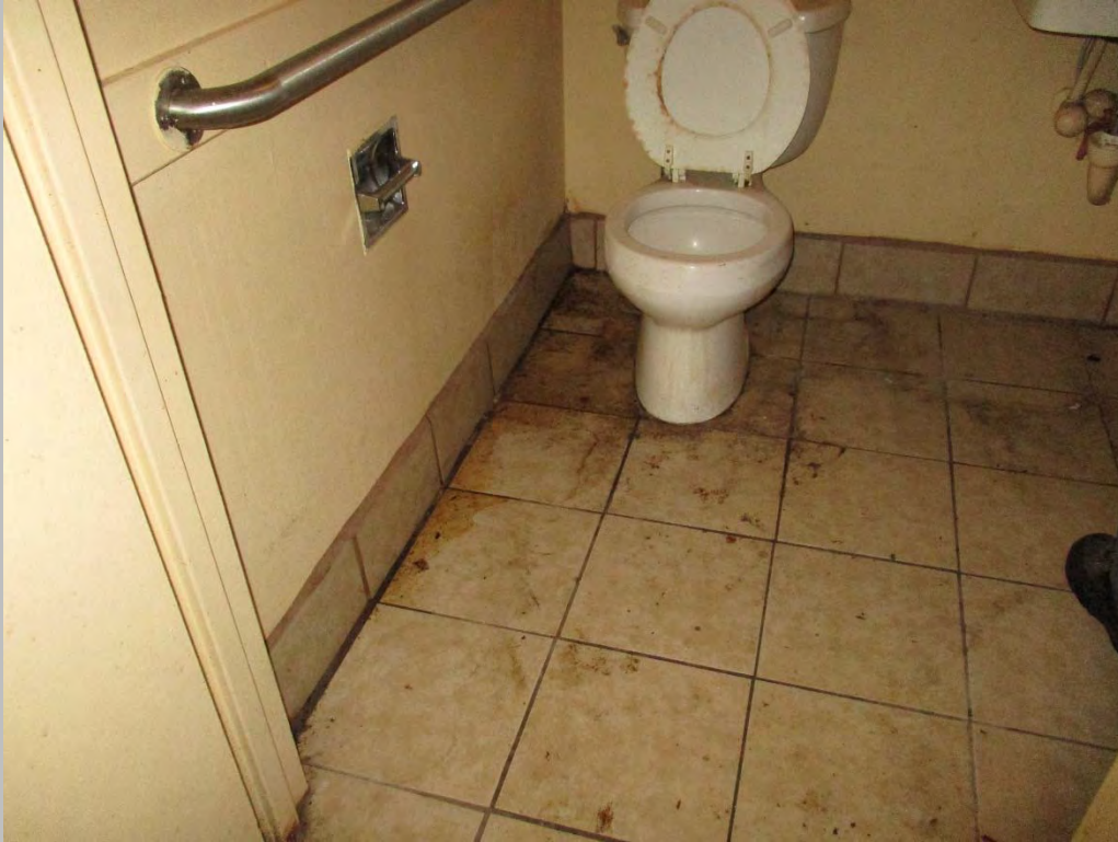
Typical dwelling unit bathroom
